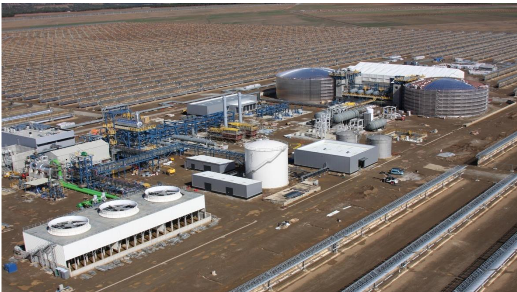
Figure D2 View of the power block in Andasol-1
