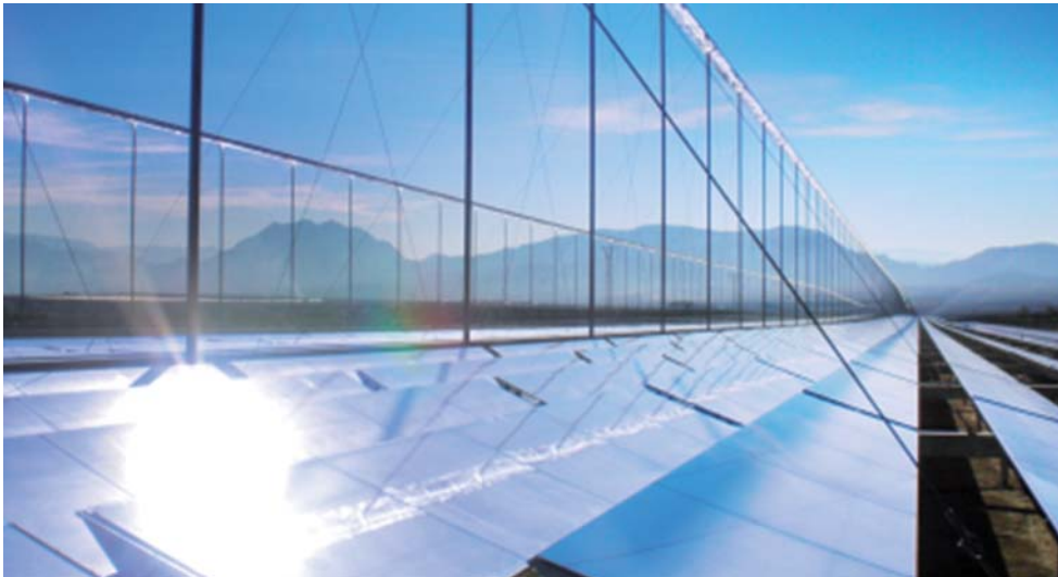
Figure 6. Power plant in Puerto Errado 1, Murcia. Majority ownership by EBL, developed by NOVATEC.
