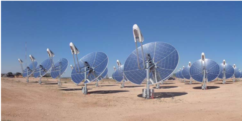
Figure 7. Power plant in Casas de los Pinos, Cuenca. Owned by Renovalia, with engines Infinia.
