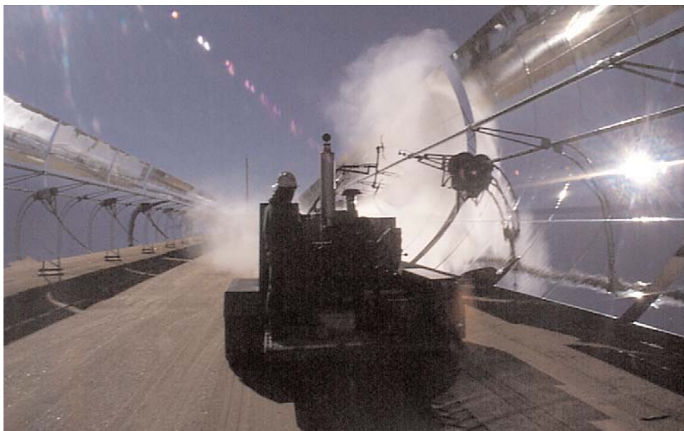
Figure 38. Mirror cleaning process in a parabolic through CSP plant.
