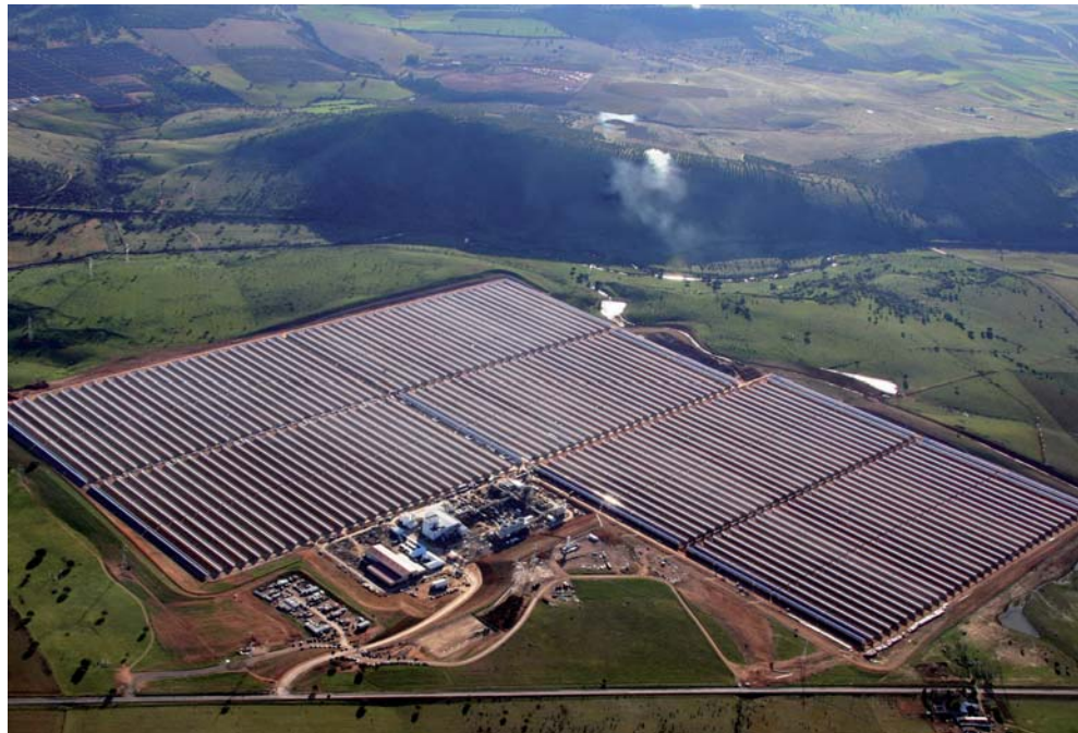
Figure 9. Power plant Ibersol Puertollano in Ciudad Real. Owned by Iberdrola.
