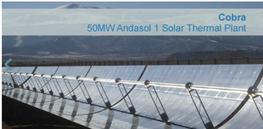
Parabolic trough: >90% of global CSP ~2011
