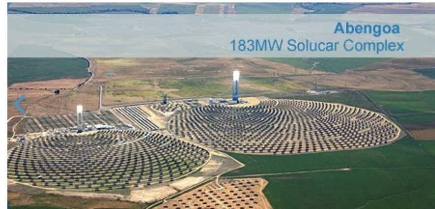
Central receiver 'power tower'
