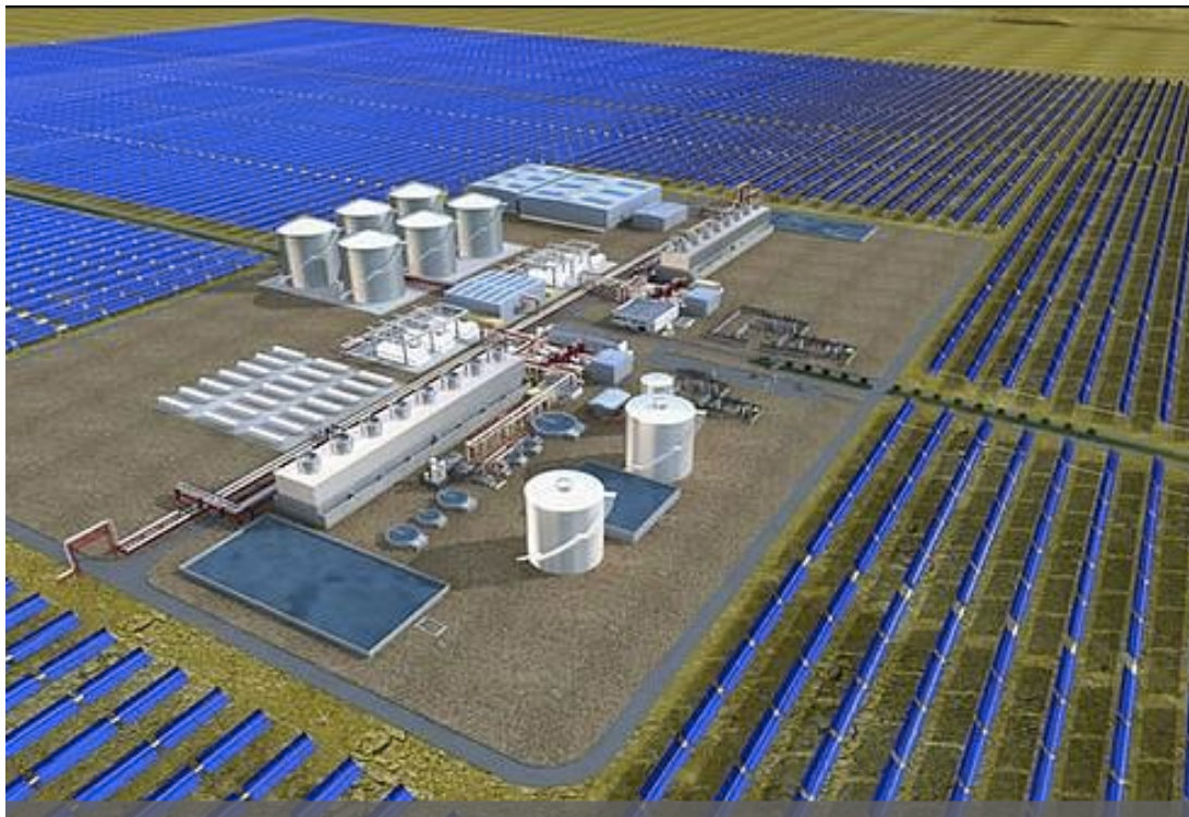
Abengoa Solar - Solana – Phoenix, Arizona, USA (under construction)
