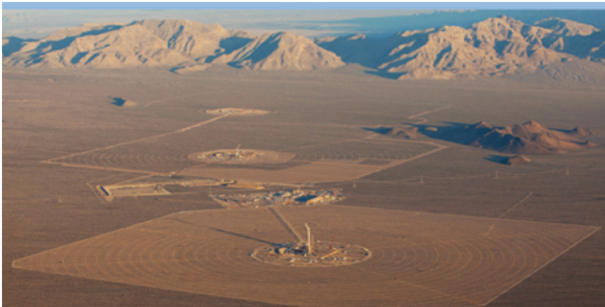
BrightSource Energy - Ivanpah SEGS – Mojave Desert, California, USA (under construction)
