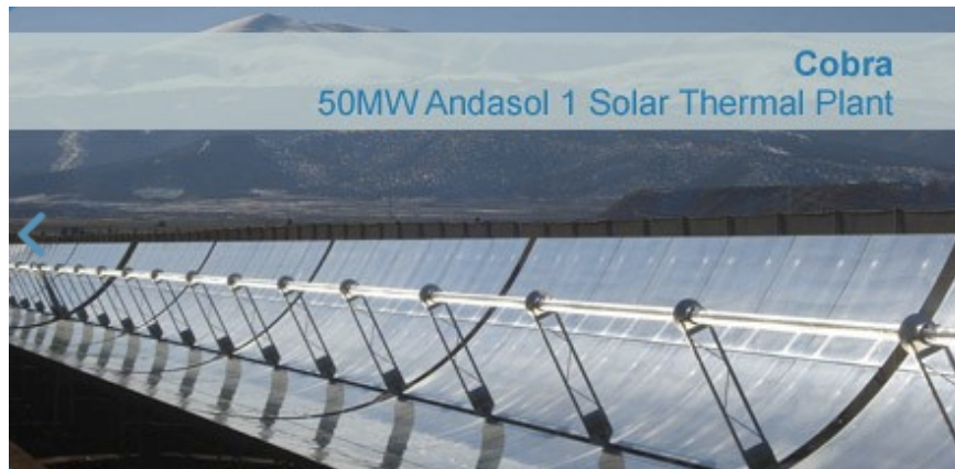
Parabolic trough: >90% of global CSP ~2011
